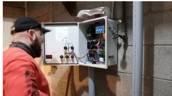
Victor Bevilacqua checks out an issue with our sump pumps.
