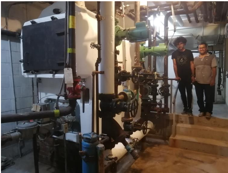
Sonny Costa Junior ( centre ) with Bruno and Alessandro , nearing the completion of the work on our Church boiler, July 2022. All the original insulation, which contained asbestos, had to be removed and replaced with fiberglass.
