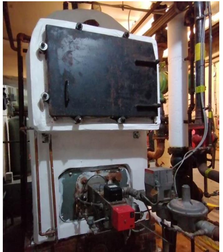
Sonny Costa Junior ( centre ) with Bruno and Alessandro , nearing the completion of the work on our Church boiler, July 2022. All the original insulation, which contained asbestos, had to be removed and replaced with fiberglass.
