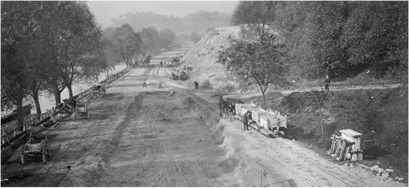
Above: The Don Roadway is built along the East side of the new Don River channel, straightened out from its natural original curving shape in the 1890's.
